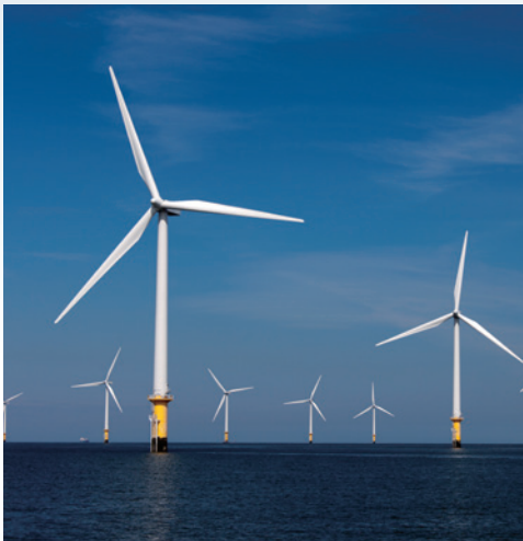
SIEMENS transformer in wind power.
