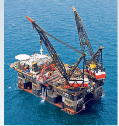
SIEMENS transformer in deepwater drilling platform.
